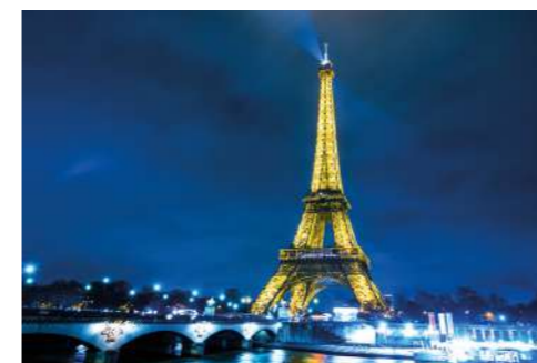
Eiffel Tower - FRANCE
